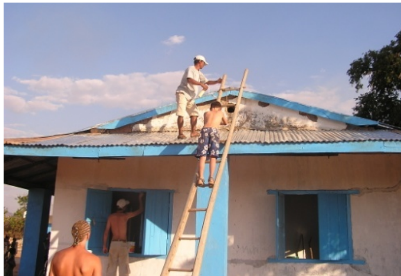
Figure 5: Rehabilitating the maternity clinic in Ankavandra
